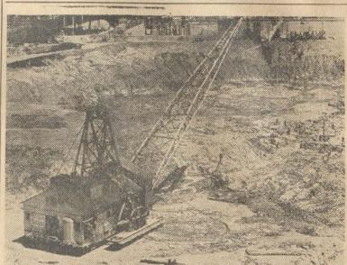
NTIL LAST NOVEMBER the area where this dragline is working was a part of the Tennessee river bed at the TVA's Kentucky Dam site. One of the greatest offer dams ever erected in dam construction encloses this area, which covers about 0 acres. This giant dragline removes six cubic yards of material at a bite.
