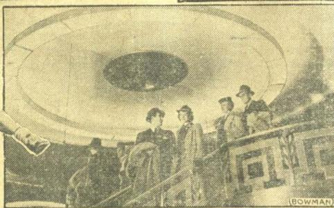
"GLASSETERIA" . . . Featuring one 120-foot wall entirely of mirrors, another of vitrolite, and plate glass stair panels, new Chicago cafeteria symbolizes "glass age" trend in building construction. Huge ceiling light shown is actually semi-circular, but is "doubled" by the mirror wall.
