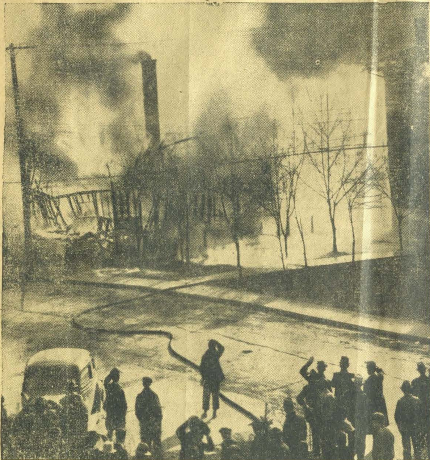
Smoke spirals from the Floyd County jail as fire in 1938 razed the Stewart Boarding House.
