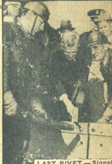
LAST RIVET —Signaling the last bit of construction work on the Golden Gate Bridge, San Francisco, the last rivet, made of gold, placed by Chief Engineer Joseph B. Strauss was driven by the crew that drove the first rivet on the job.
