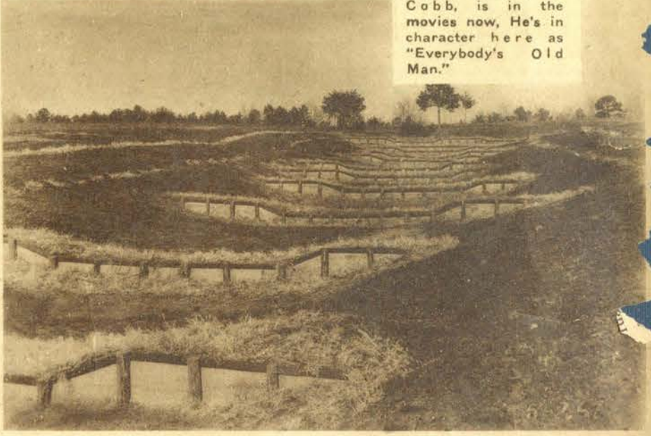
ON THE OTHER HAND is demonstrated the steps necessary to treat a gully near Spartanburg, South Carolina. Check dams are installed, the banks of the gully sloped and planted. Wire and straw are placed in the dams to catch surface soil washed down the gully. (Soil Conservation Service Photo.)
