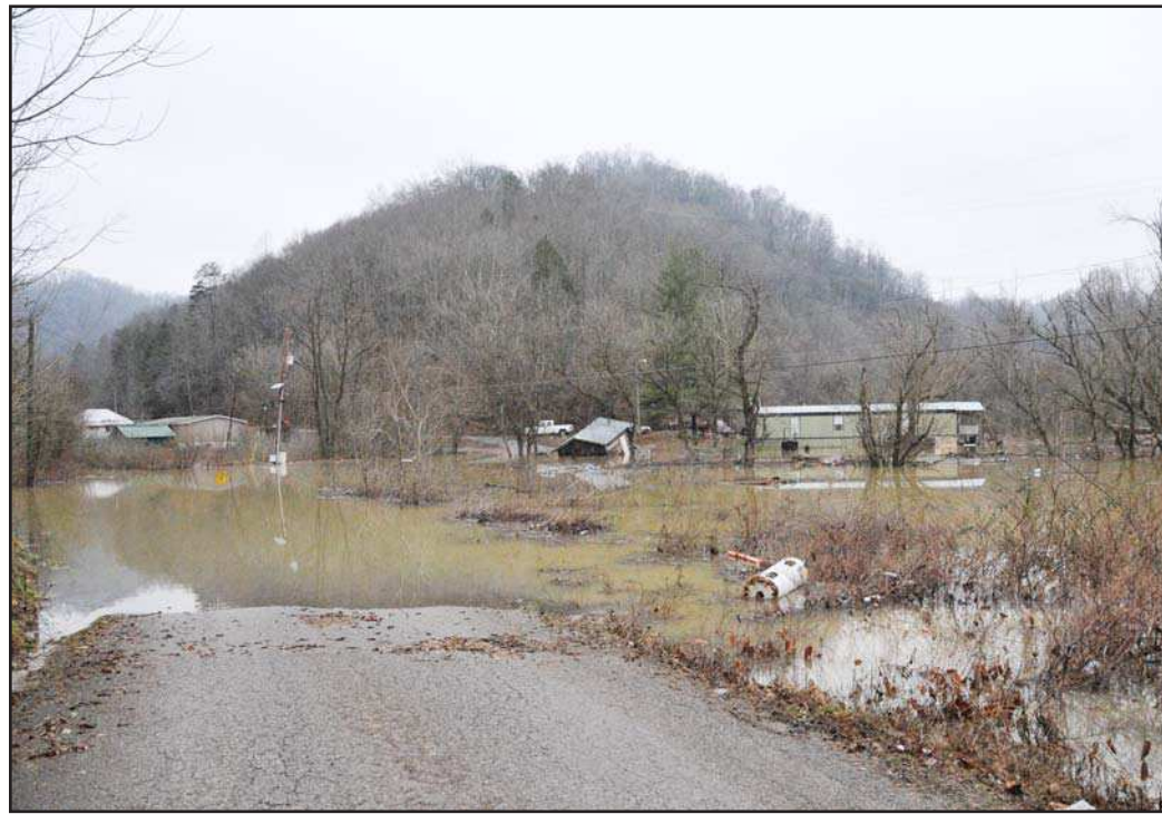
Floyd Chronicle photo by Mary Meadows A structure was washed off its foundation after flooding on Oklahoma Hollow in Allen this weekend. A mobile home near this location was surrounded by water on Feb. 12.
