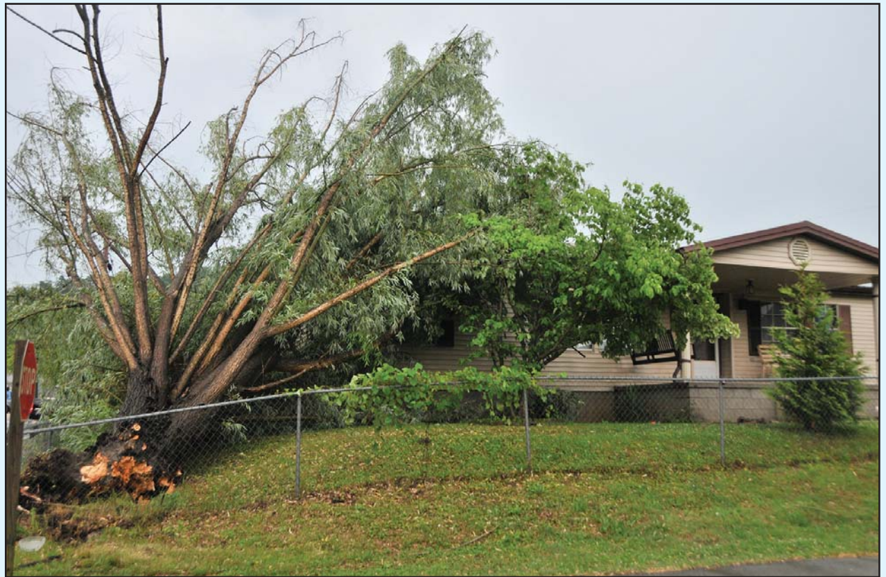
A large tree fell on this home, located at the corner of Main Street and Stanley Street in West Prestonsburg Wednesday, causing a power outage in the neighborhood.
