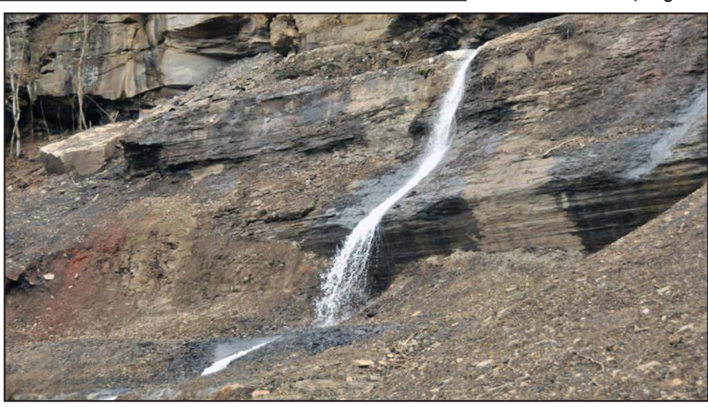
Floyd Chronicle and Times photo by Mary Meadows The Division of Abandoned Mine Lands is rehabilitating an old coal mine site near Ky. 1086 in Wayland. Once the work is complete, city officials hope to construct a park area with river access across the road from this site.
